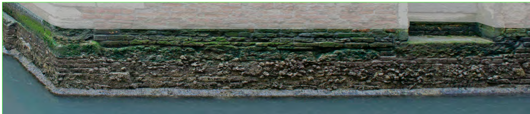
Fig. 27. Upper portion of Venetian Substructure Complex , brick strata, in-situ.
