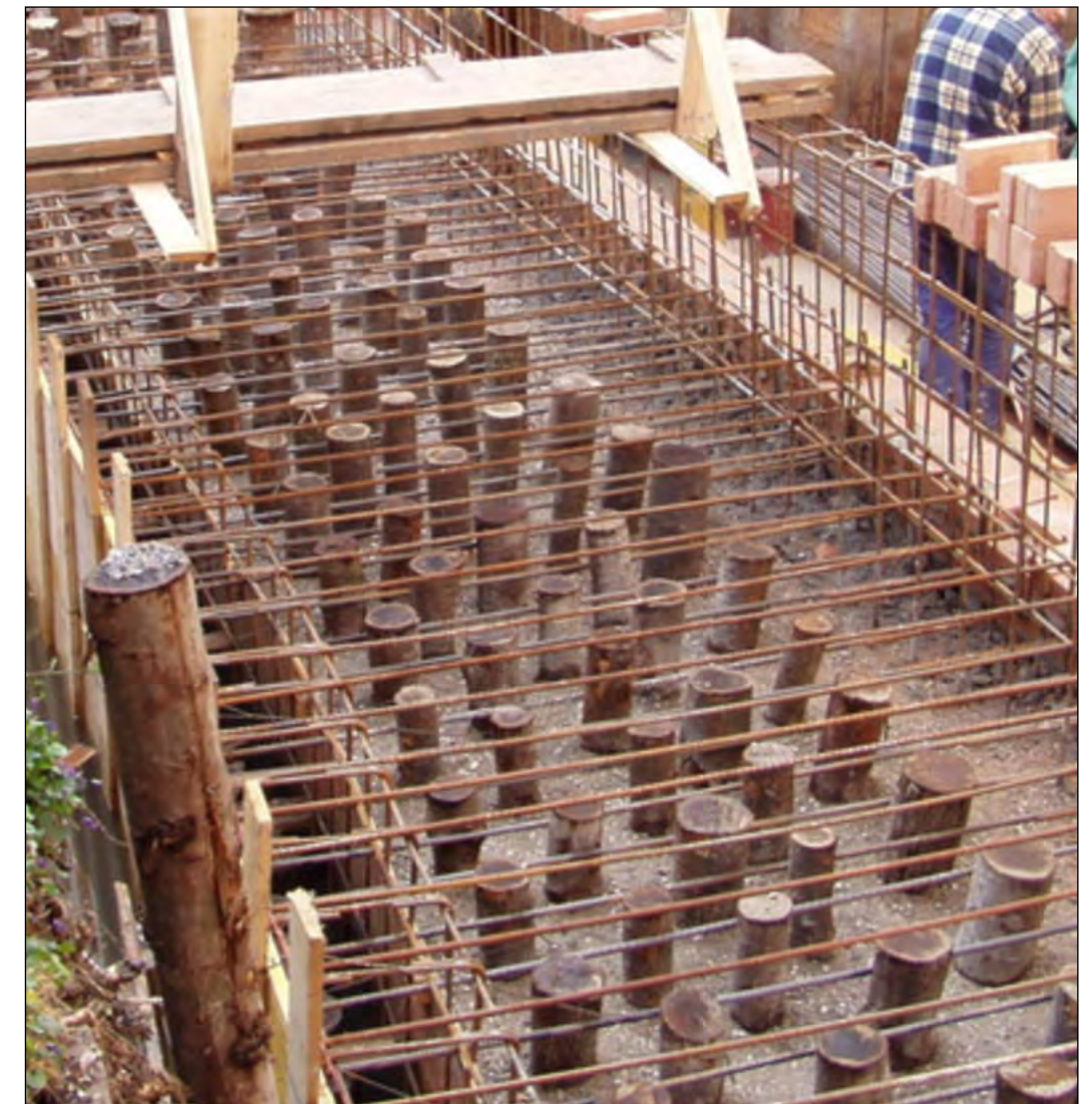
Fig. 20. Excavation and repair of a site in Venice, showing foundation pilings. Allo Squero, Venice, It.
